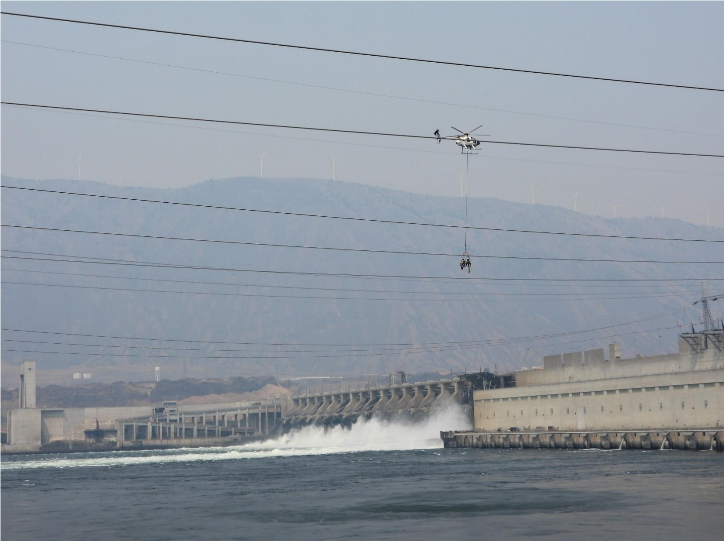
BPA Line Repair
