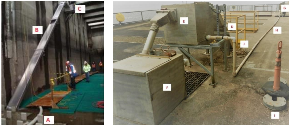
Figure 4: Images of the north fish ladder (NFL) lamprey passage system (LPS) (*Note* the first picture is facing east, and the second picture is facing west): (A) bollard field (B) access ramp (C) resting box (D) ramp entering the upwelling box (E) upwelling box (F) holding tank (G) lamprey pumps (H) water supply line (I) pump location from the 2019 modification (J) pneumatic airlines to flush the rest box.
