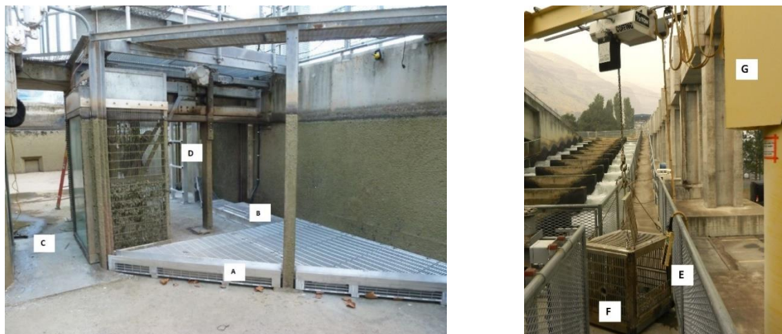
Figure 5: Images of the south fish ladder (SFL) lamprey trap system (LTS): (A) entrance (B) diversion conduit (C) count station window/crowder (D) trap box guide (E) trap box (with access hatch removed) (F) lamprey entrance port (G) trap hoisting jib crane. *Note* when in operation picketed leads rest atop the LTS entrance (A), and upriver from the trap box guide (D). These picketed leads guide fish to the count station window (D).
